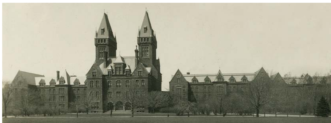
Historic Buffalo State Hospital buildings, circa 1900 (Source: Goody Clancy 2009)
