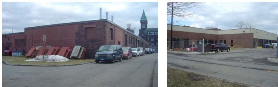
BPC and BSC Maintenance Facilities
