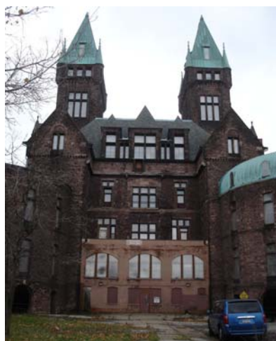
1927 rear addition to Building 45 (Source: Goody Clancy 2009)
